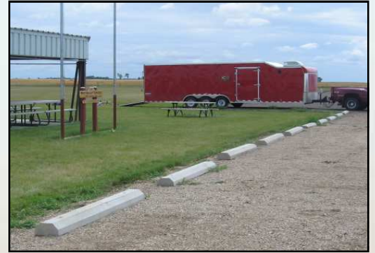
Concrete parking markers replaced the deteriorating rail road ties....
